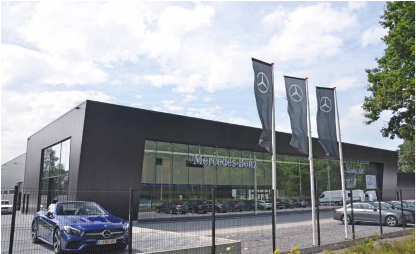
This car dealership in Belgium has been fitted with a rooftop PV array by Intellisol, which won the contract by using intelligent modeling analysis to calculate the exact size of the solar system required.
